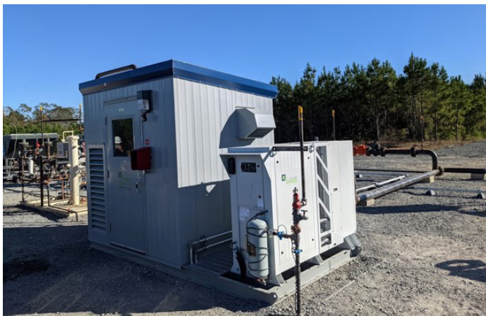
Figure 3. Qnergy CAP3 deployment in Louisiana, US. The change from natural gas to compressed air can eliminate 98% of well pad emissions.
