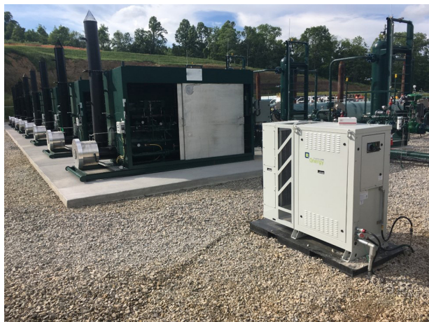
Figure 1. Qnergy PowerGen – a Free Piston Stirling Engine remote power system on a natural gas wellsite.
