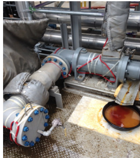
Figure 2: Compressor lube oil system before installation.
